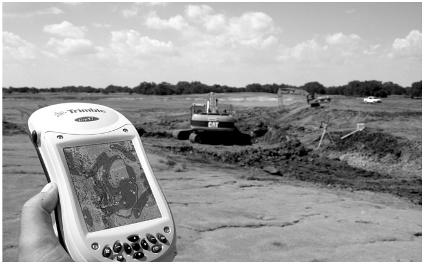
A handheld GPS receiver was integral to the design, documentation and implementation stages of the construction of Wolf Point Club in Port Lavaca, Texas.
